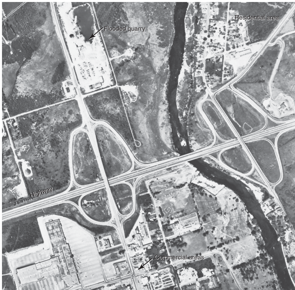
FIGURE 1-2 Aerial photograph of same property after development
